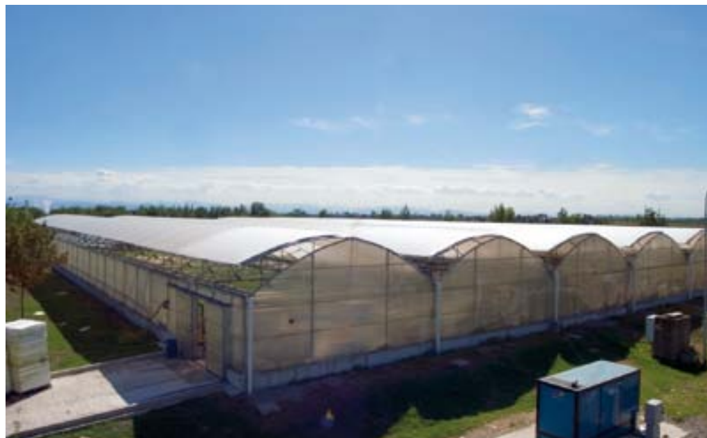
Serre alimentate a biogas
